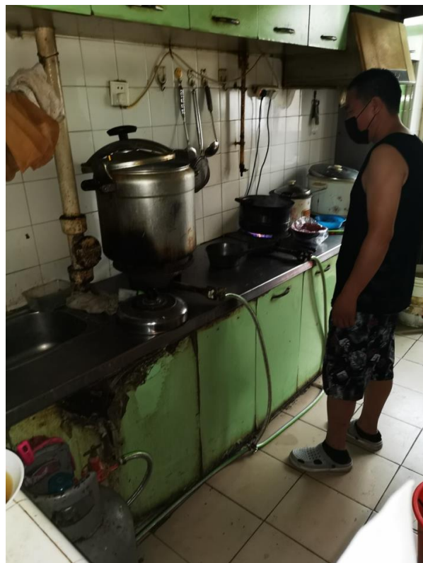
NO.6 软管穿墙
